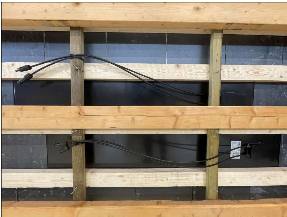
Figure 4 – Backside of test specimen, electric wiring.
